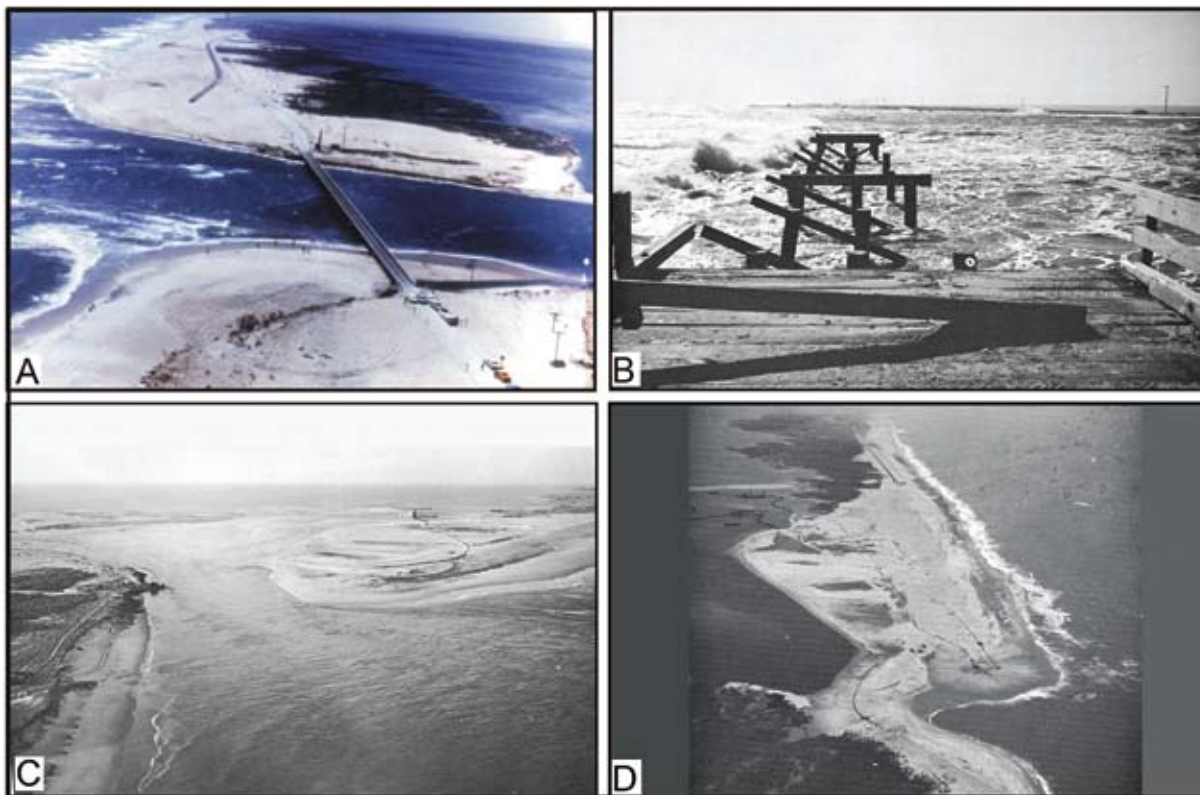
Figure 15. (A) Buxton Inlet as it appeared following construction of the Highway 12 bridge shortly after opening in 1962 (photograph courtesy of National Park Service Archives at Cape Hatteras National Park, Manteo). (B) A photograph of Buxton Inlet following destruction of the bridge during a nor'easter in December, 1962 (USACE, 1963). (C) An oblique aerial photograph of Buxton Inlet in 1963 showing the dredging and filling operation; note the pipeline feeding sand to the beach from dredging operations in the sound (USACE, 1963). (D) An oblique aerial photograph showing the Buxton Inlet location following inlet closure by the USACE (USACE, 1963).
